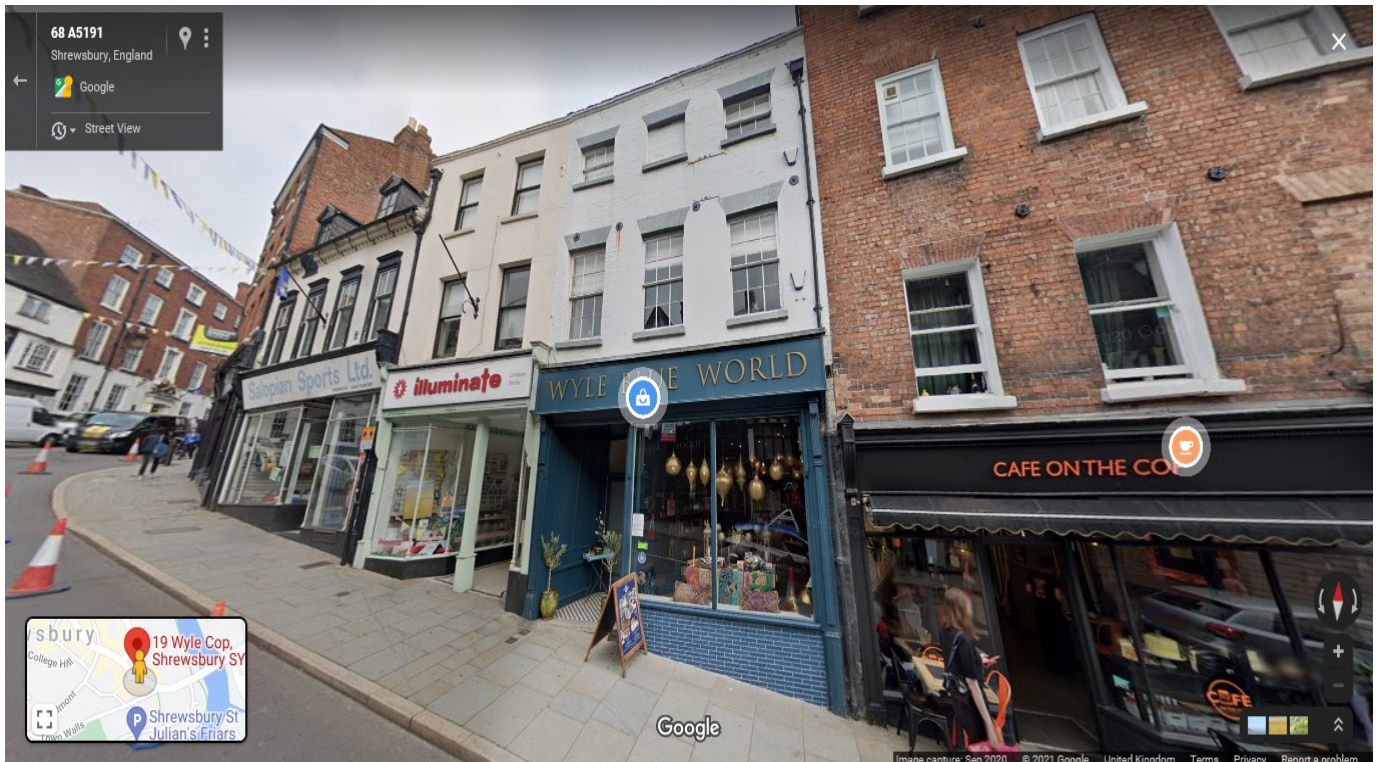
- Front view of the premises -
